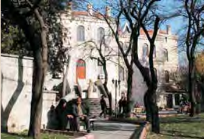
The former girls' school building today: SEV Gaziantep American Hospital's Polyclinic B Block.
